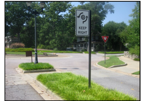
This neighborhood roundabout eases the flow of traffic by eliminating stop signs while giving added protection for pedestrians.
